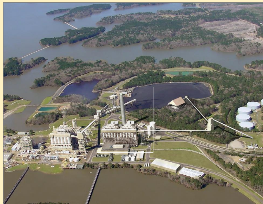
Rodemacher Power Station with Unit 3
