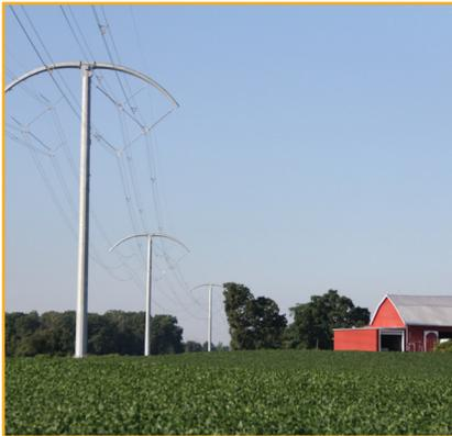
AEP Indiana Michigan Transmission Company's Sorenson – Robison Park 345/138-kV transmission line in Fort Wayne, Indiana, is the first of its kind using AEP's Break-through Overhead Line Design (BOLD®) technology. This 22-mile line, rebuilt in the existing right-of-way, provides enhanced reliability by reducing low-voltage situations and overloaded lines in the area brought on by the retirement of a significant amount of fossil generation.
